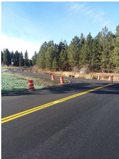
Temporary Paving is in and the Striping is Complete
