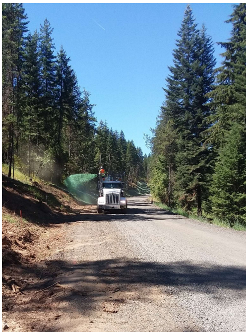
Hydra Applied Erosion Control on Kidd Island Road
