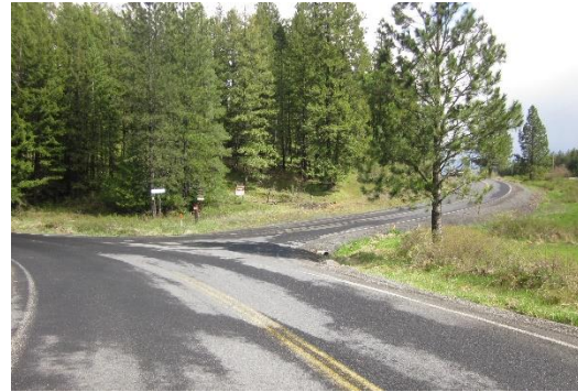
Kidd Island Road and Valhalla Road Intersection
